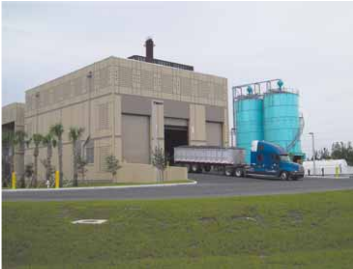
Photo 3 - SWA Pelletizer Facility
